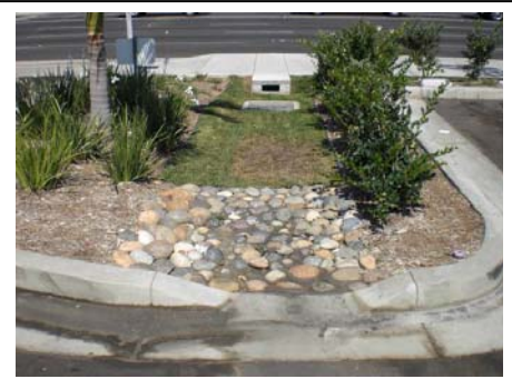
Inlet Structure Downey, CA
