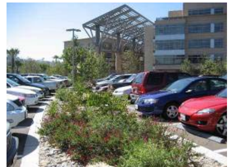
Bioretention Cell Caltrans Headquarter San Diego, CA
