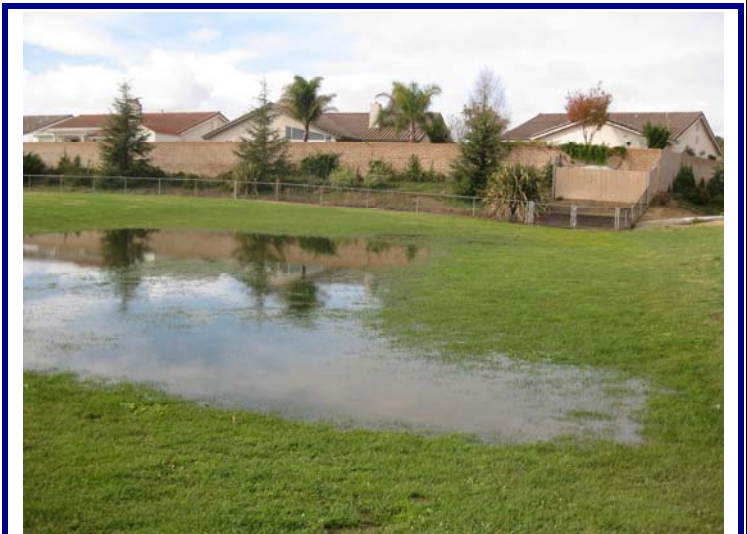
Sierra Vista Park and Storm Water Basin
