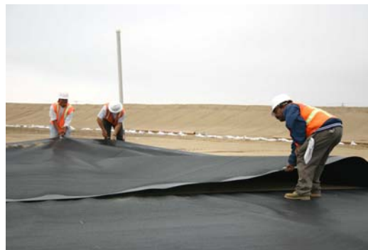
Photos: Liner being installed in mid-September, 2006, at the Santa Maria Regional Landfill. The synthetic liner is about 3/32 nd s of an inch thick. NHIS will be deposited on top of this layer.
