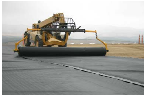
Photos: Liner being installed in mid-September, 2006, at the Santa Maria Regional Landfill. The synthetic liner is about 3/32 nd s of an inch thick. NHIS will be deposited on top of this layer.
